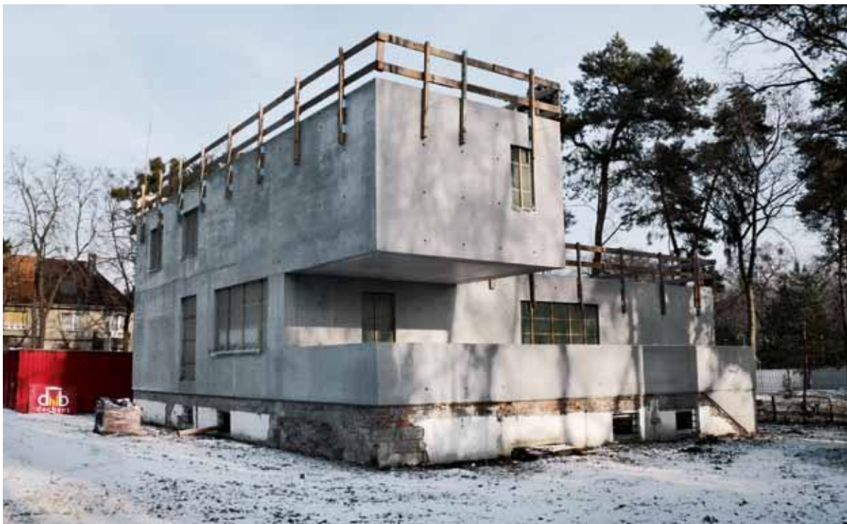
Gropius House, south side view, 2012
